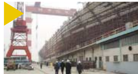
The shipyard has a large container ship, 190 metres long, under construction.
